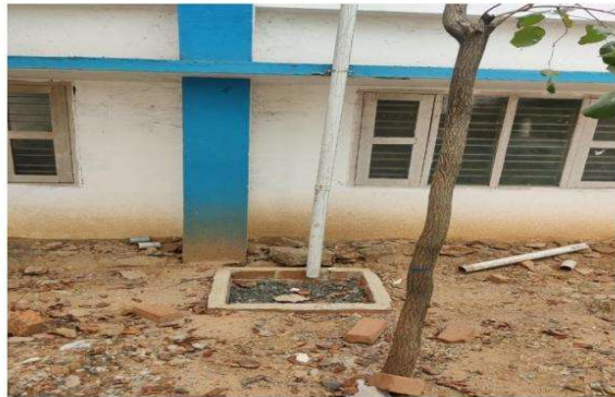
Rain Water Harvesting Implemented inside the campus
